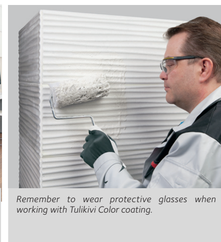
When the coating has dried, replace the doors. Your Tulikivi fireplace is now as good as new! Remember to allow the surface to dry for one week before using the fireplace again.
